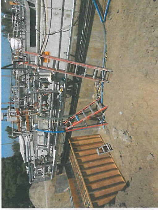
Chlorine Contact Basin Outfall Structure and Installation of Duct Bank
