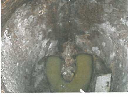
Ramona Corroded Siphon Manhole
