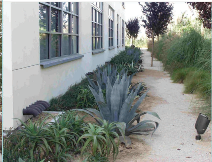
Rain from the roof of this commercial structure drains into the plant beds below.
