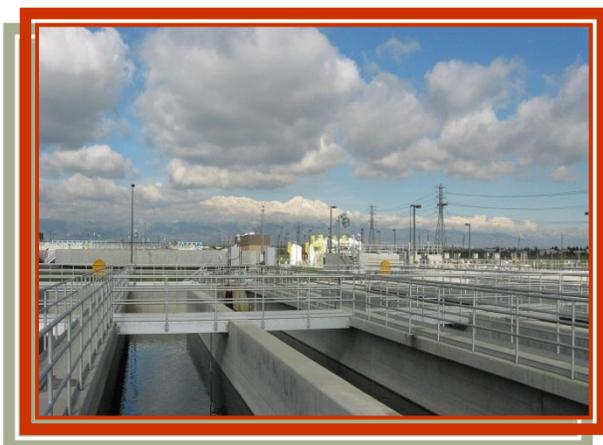
RP-5 is located in the Southwestern area of the Agency's boundary in the City of Chino. This facility was originally commissioned in 2000. RP-5 treats an average flow of approximately 8 mgd. RP-5 includes several treatment processes that contribute to providing a quality recycle water pursuant to the State of California Title 22 regulations.
