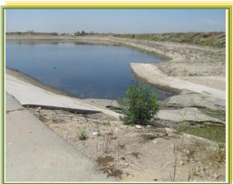
The Turner Basins are capable of receiving up to 10 cubic feet per second of recycled water flow for ground water recharge. The basin improvement projects will enable the full recharge capacity of the basins.
