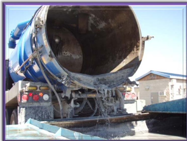
Pipeline Cleaning Discharge – IEUA Vactor Truck
