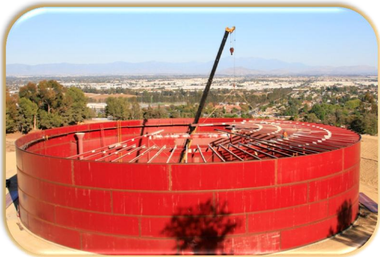
930 Zone Reservoir Installation of Roof Panels
