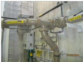
Primary Sludge piping and pipe fittings appear to be in good condition with no signs of corrosion.
