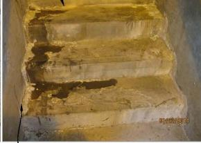
The leaky joints between stairs and the concrete wall appear to have had polyurethane injection. It is not apparent if the leak has been stopped. The application methodology and workmanship is questionable. RMS recommended Howard Ridley Company (HRC) in Chino, CA (909) 590-7415 to CCWRF plant staff.
