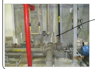
Leaky crack in lower portion of the pump room east wall.
