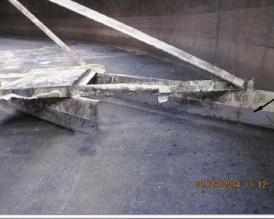
Scraper Blade. The protective coating on majority of the blades has delaminated. However, there was no signs of metal corrosion.
