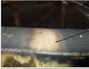
Rake Arm assembly, upper chord. We wire brushed the top surface and the coating emerged. The protective coating appears to be in good condition.
