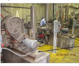
Primary Sludge piston pumps: These are older pumps with many moving parts and according to operations staff they require frequent maintenance. There could be safety issues involved with this heavy maintenance
