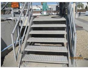
The galvanized steel stair and its handrails and grated treads to the motor and control deck is in good condition with no visible signs of corrosion.
