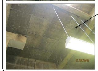
Primary Sludge pump room concrete roof appears to be in good condition with no signs of rebar corrosion or concrete deterioration No signs of corroded reinforcing steel was noticed.
