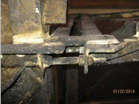
Cross ties between the rake arm assemblies appears to be in good condition, with no visible signs of corrosion.
