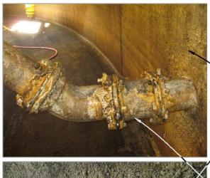
The metal corrosion, due to coating failure, is on the surface only and it has had no significant affect on the strength of the piping, pipe flanges or the connection bolts.
