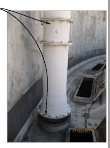
Foul air ducting, duct supports and the scrubber system shown no signs of any significant corrosion or deterioration.
