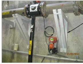
Primary Sludge piping supports appear to be in good condition with no signs of corrosion.
