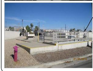
Concrete deck around the pump room stairway access. The 3-line galvanized steel railing and the kick plates show no signs of corrosion.
