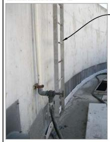
Ladder to lower deck is galvanized and it is in good condition. The Ladder rungs are not serrated and do not comply to current OSHA safety requirements.
