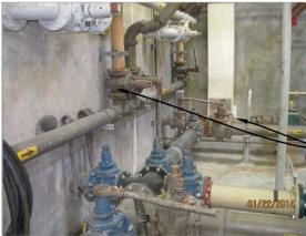
Minor surface corrosion was noticed on some of the valves and fittings in the pump room.
