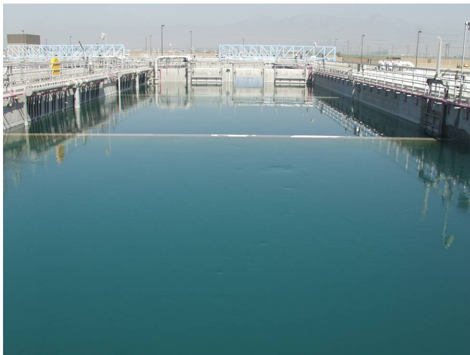
Regional Plant No. 5
