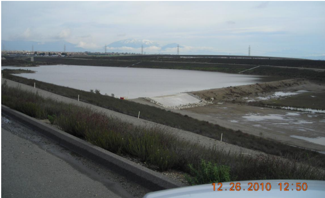
San Sevaine 5 with newly installed hardened spill point in conservation berm
