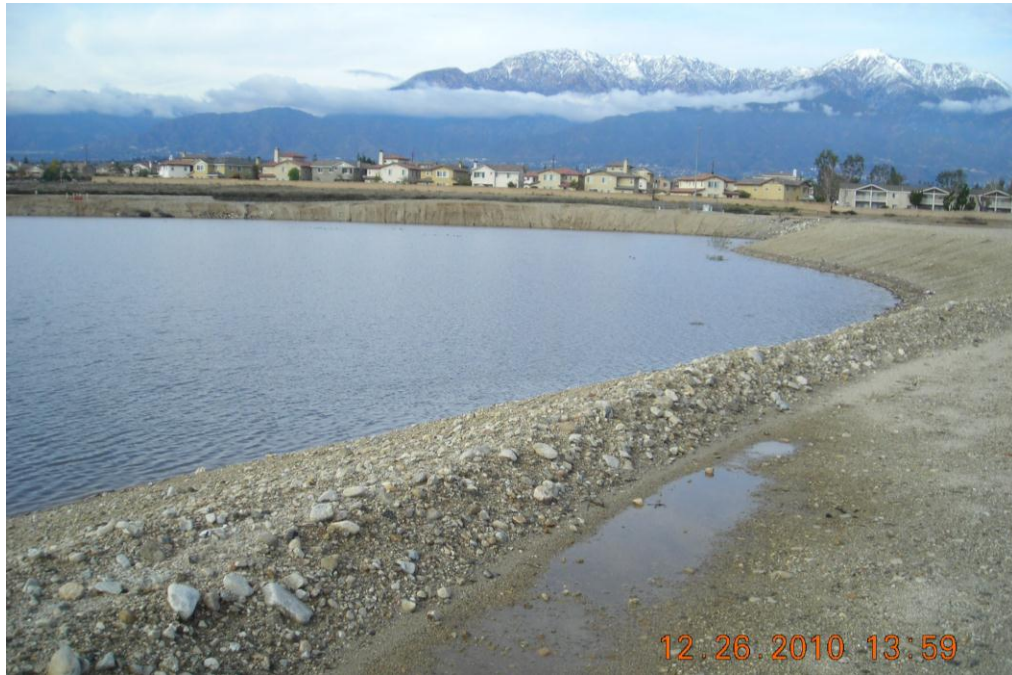
Turner Basin 4 at Capacity
