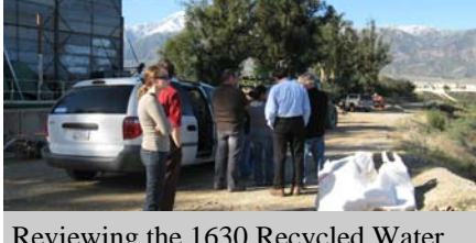
Reviewing the 1630 Recycled Water Pipeline Installation at Victoria Basin.
