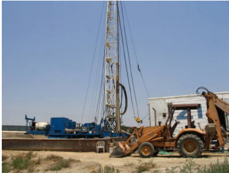
Drilling Monitoring Well II-MW-2
