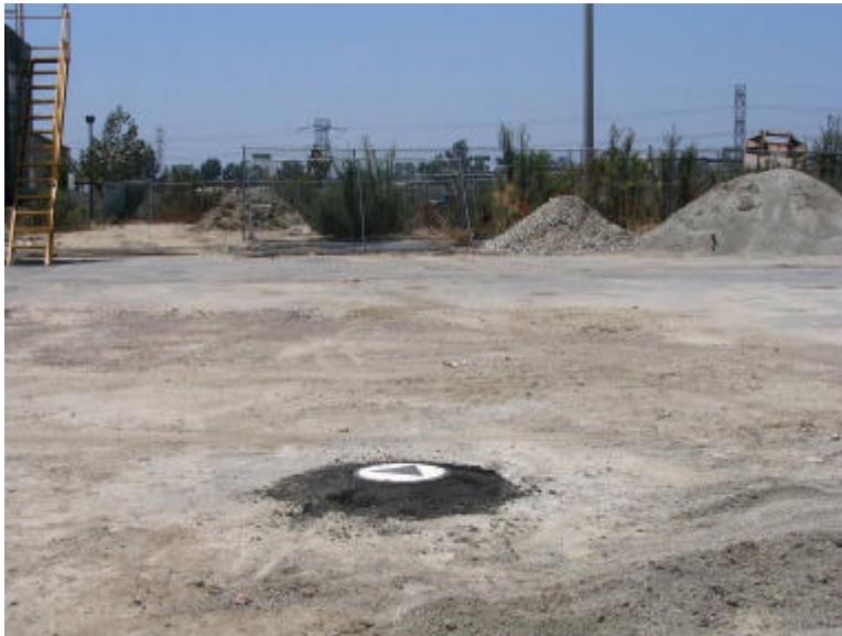
Drilled Monitoring Well II-MW-1
