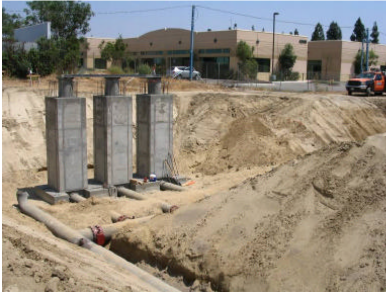
Excavation Pit with the Three Pump Cans
