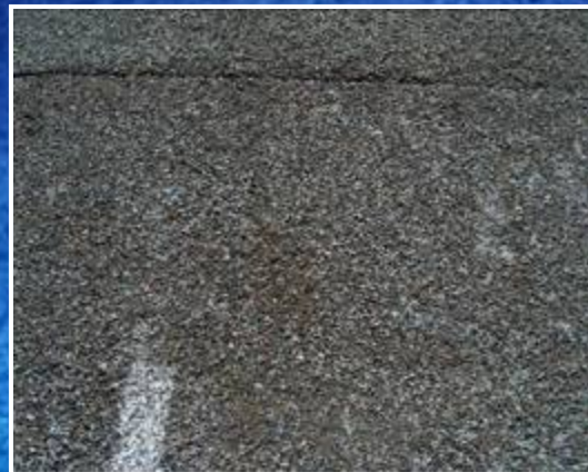
Pervious Concrete = 12,000 Sq. ft
